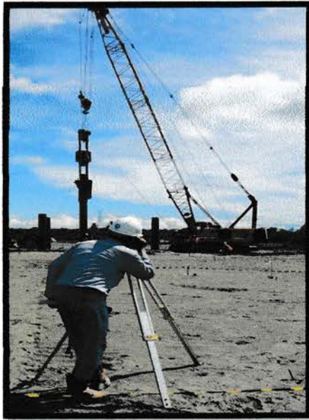
Gambar 4. Surveying dan alat survey (Total Station)
