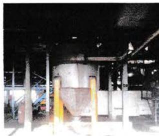
**Gambar 3.4. *Sand Trap Tank***
