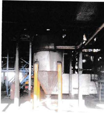
**Gambar 3.18. *Sand Trap Tank***
