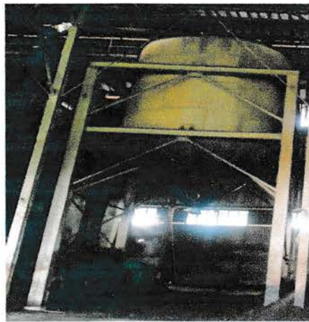
Gambar 3.63 Bunker Inti Sawit
