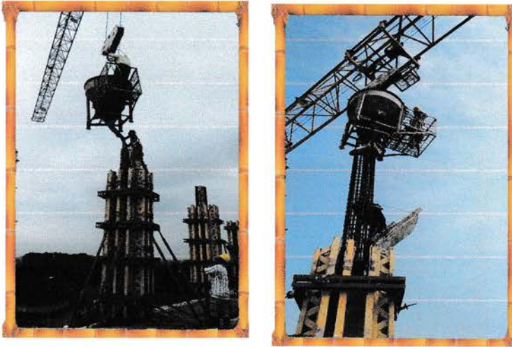
Gambar III.21 Proses pengecoran
