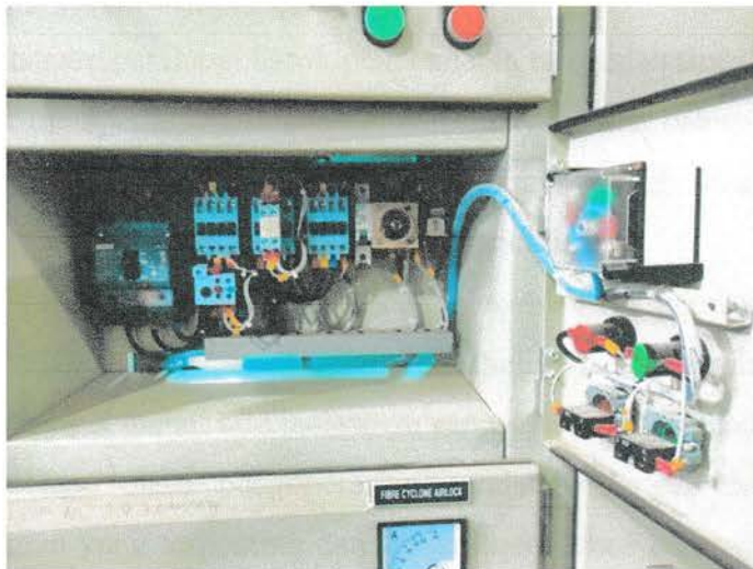
Gambar 2.15 CT (current Transformator)
