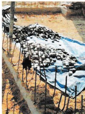
Gambar 6. a Beton Decking
