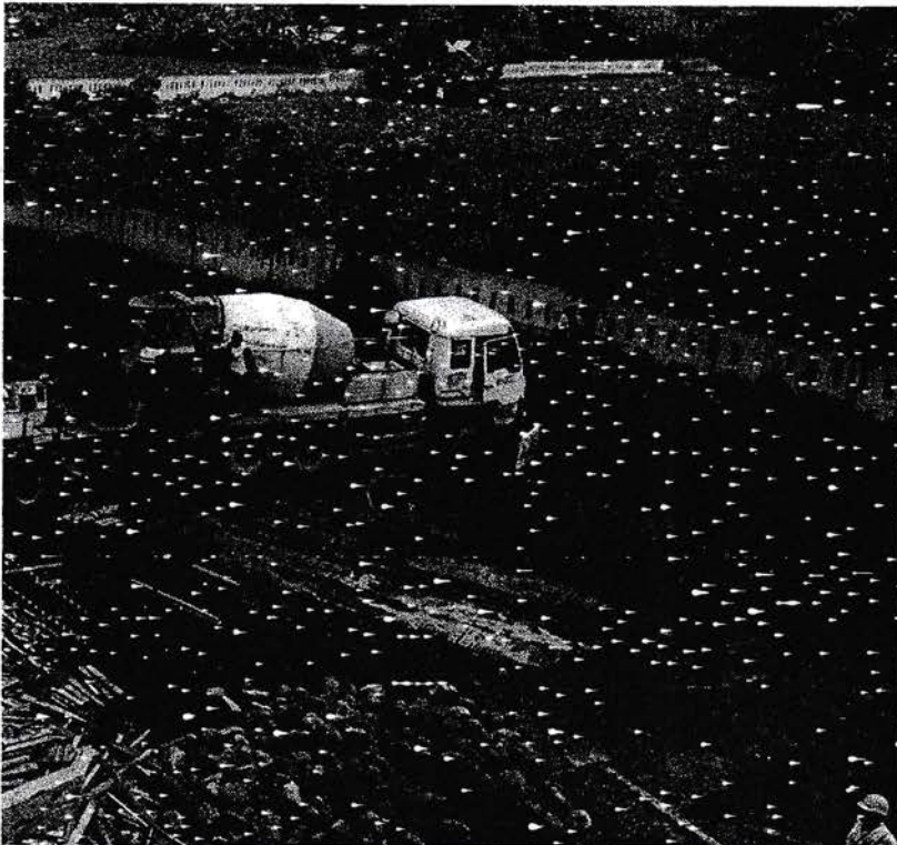
Gambar 3.16. Beton ready mix
