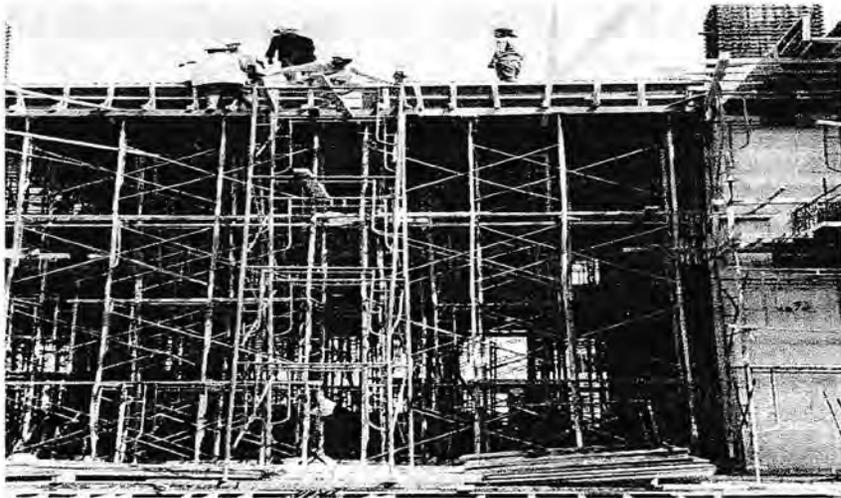
Gambar 3.14 Bekisting balok
