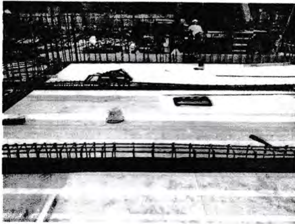
Gambar 3.16 Bekisting plat lantai
