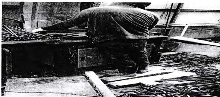
Gambar 3.5 Bar Bending
