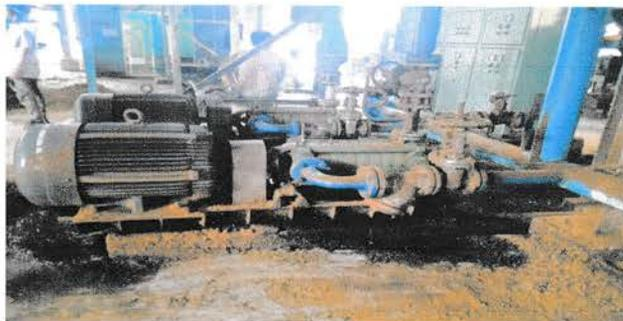
**Gambar 3.29** *Electric Feed Water Pump*
