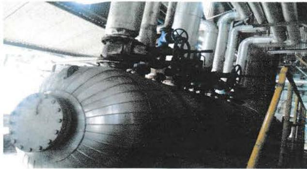
**Gambar 3.39 Back Pressure Vessel (BPV)**
