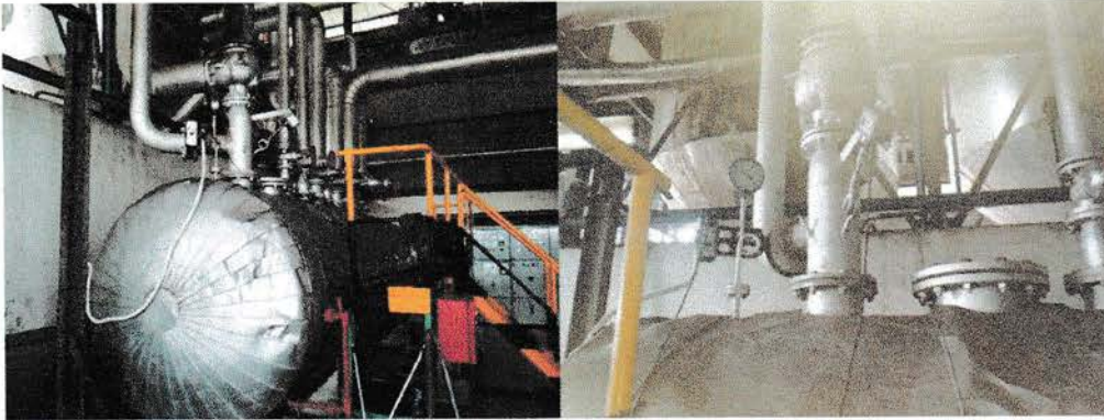
Gambar 4.5. tabung BPV ( break pressure vassel )
