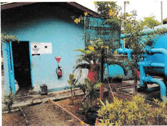
Gambar 4.1 Water treatment plant
