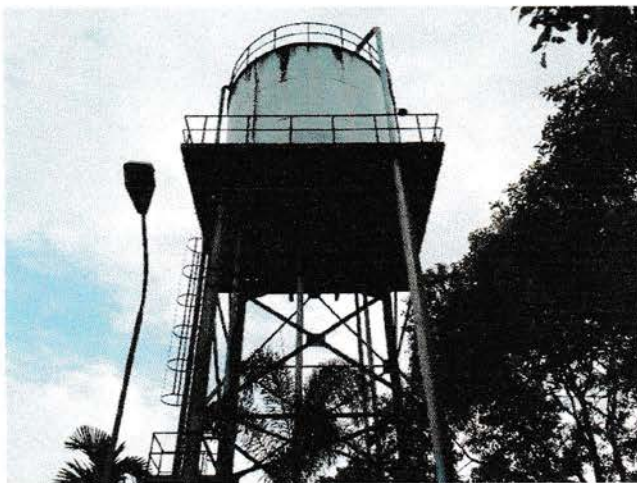
Gambar 4.1.5.a water tower tank
