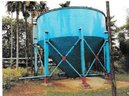
Gambar 4.1.2 clarifier tank
