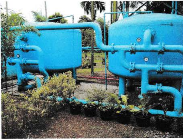
Gambar 4.1.4 sand filter
