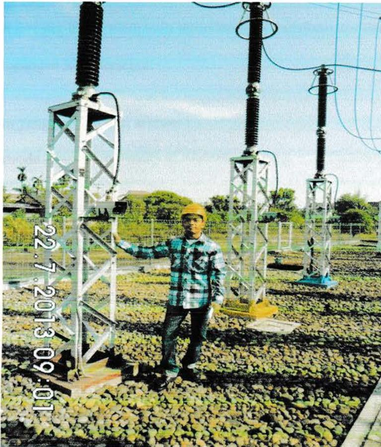
Gambar II – I : Lightning Arrester
