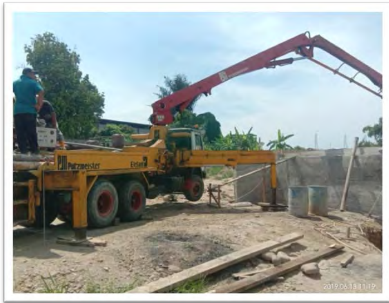
Gambar 2.13 Concrete pump
