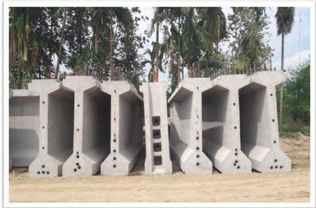
Gambar 2.11 Balok Girder I
