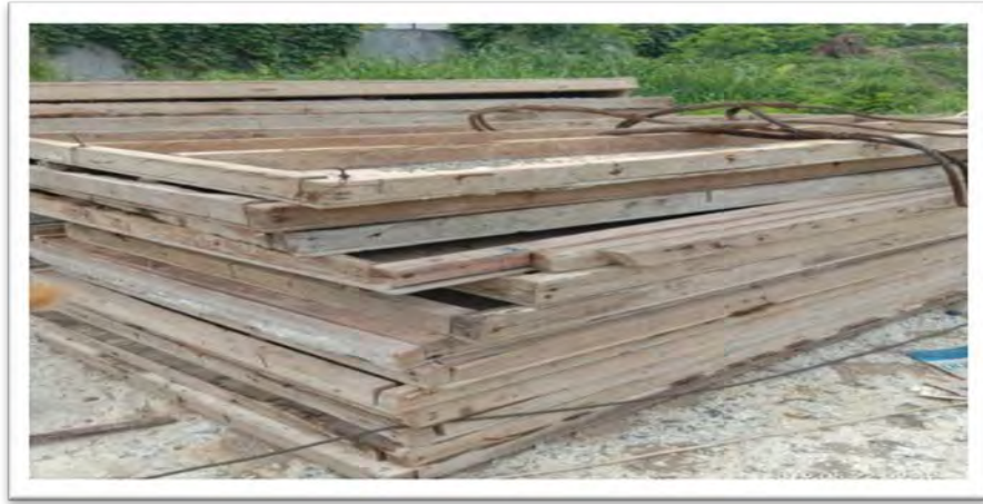
Gambar 2.15 Bekisting Konvensional (Bekisting Tradisional)
