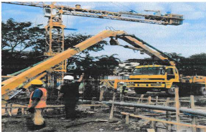
Gambar 3.2.2 Concrete Pump
