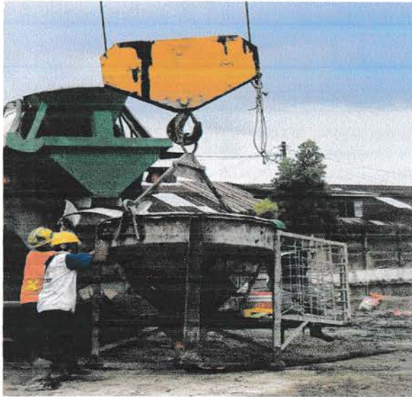
Gambar 3.2.15 Concrete Bucket
