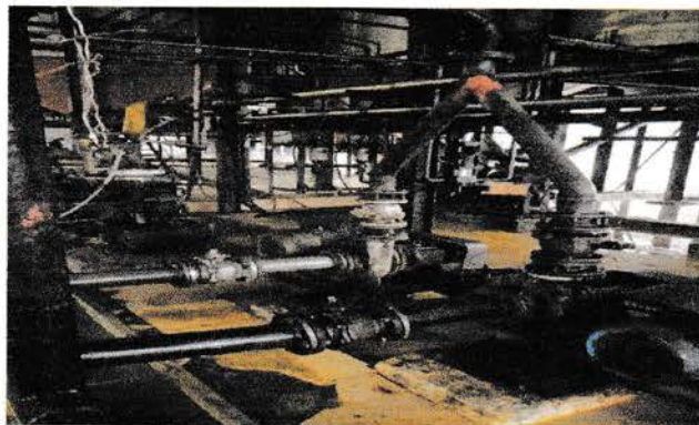
Gambar 3.26 Oil Transfer Pump
