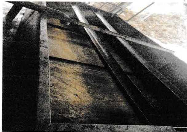
Gambar 3.18 Crude Oil Tank
