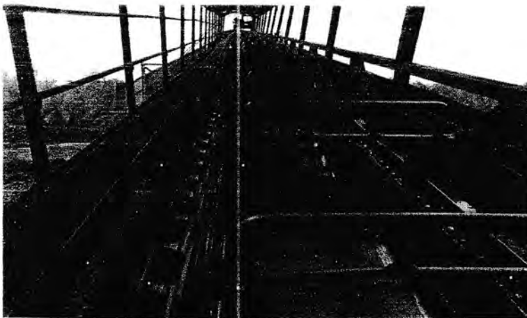
Gambar 3.11. Empty Bunch Conveyor
