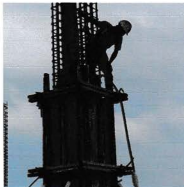
Gambar 4.44 Proses Perataan Cairan Beton
