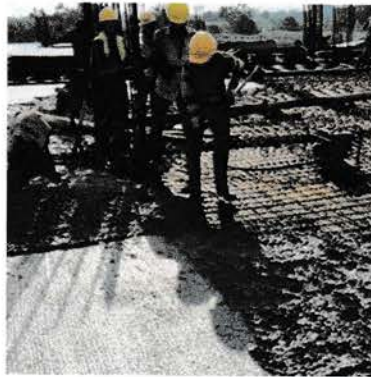
Gambar 4.53 Proses Pengecoran
