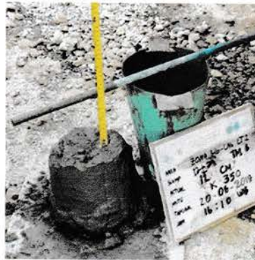
Gambar 4.59 Proses Slump Test
