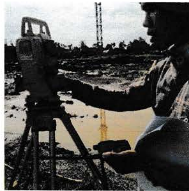
Gambar 4.26 Penentuan As Tie Beam menggunakan Total Station
