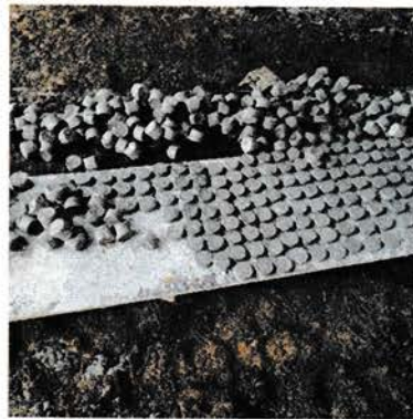
Gambar 4.19 Beton Decking
