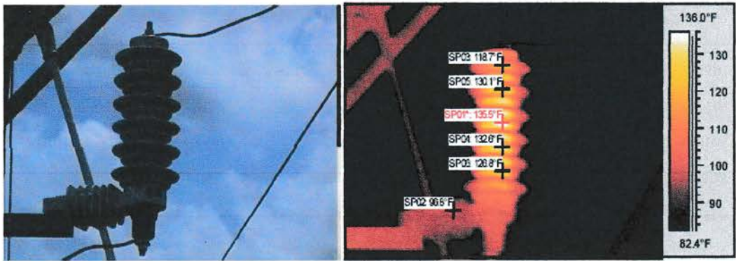
Gambar 3.1 Lightning Arrester
