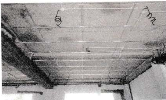
Gambar III.4 Rangka Metal furing
