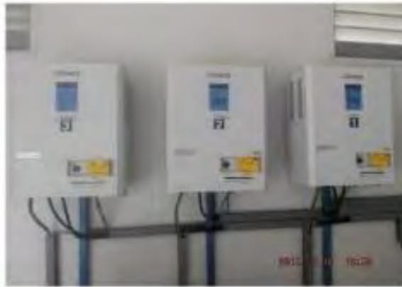
Gambar 2. 7 Solar Charge Controller
