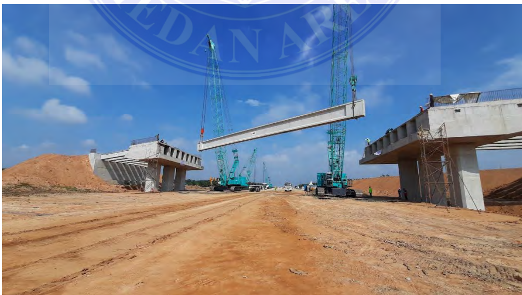
Proses Erection Girder
