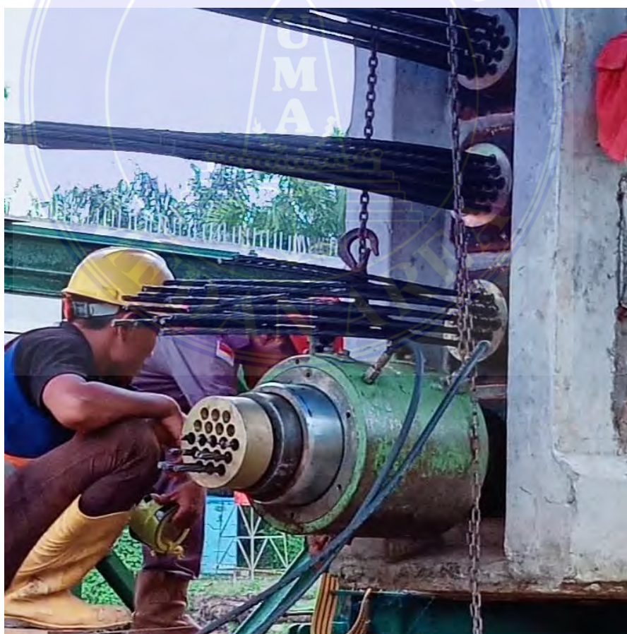
Proses Stressing Girder
