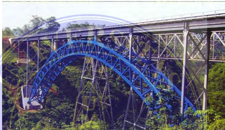
Gambar 2.25 Jembatan rangka Sumber: Cable Stayed Bridges (1999)
