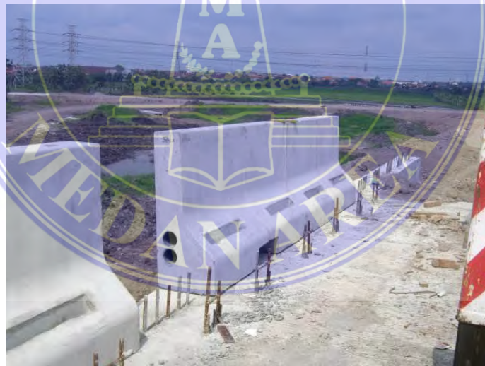
Gambar 2.1 Barrier/Parapet Sumber: PT. CALVARY ABADI
