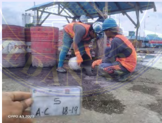
Gambar 3.8 Grouting Sumber : dok. PT. Artek Utama Consultant
