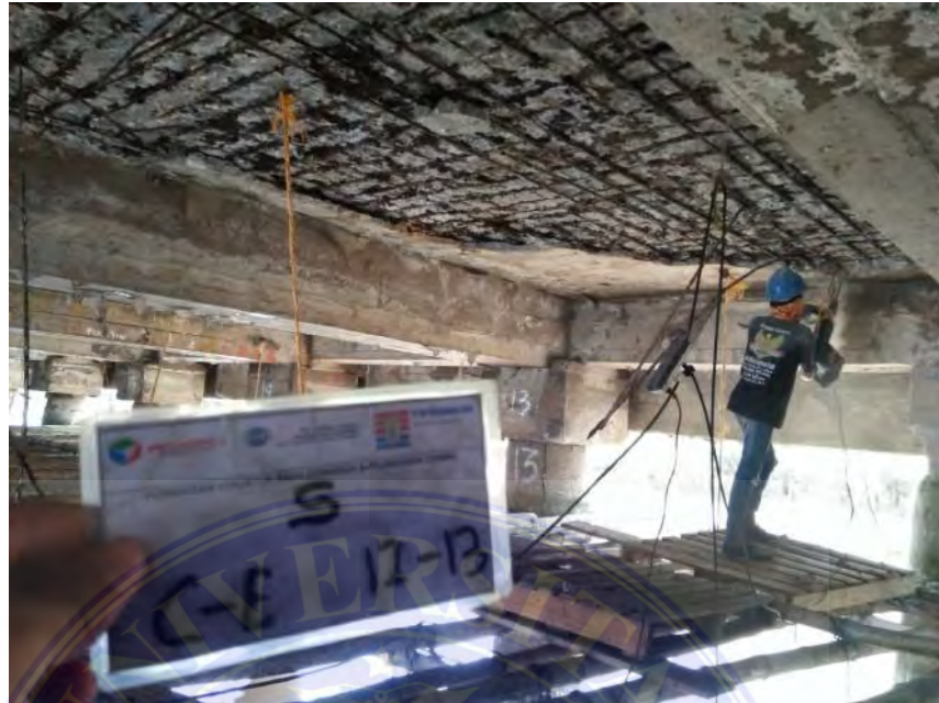
Gambar 3.5 Chipping Beton Sumber : dok. PT. Artek Utama Consultant
