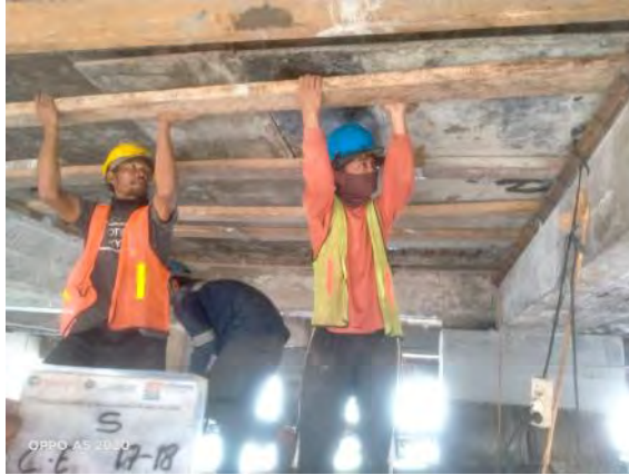
Gambar 3.7 Bekisting Sumber : dok. PT. Artek Utama Consultant
