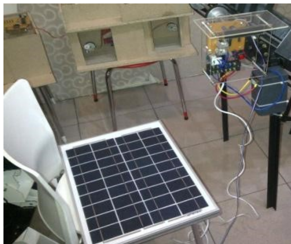
Figure 3.3 Solar Cell Installation
