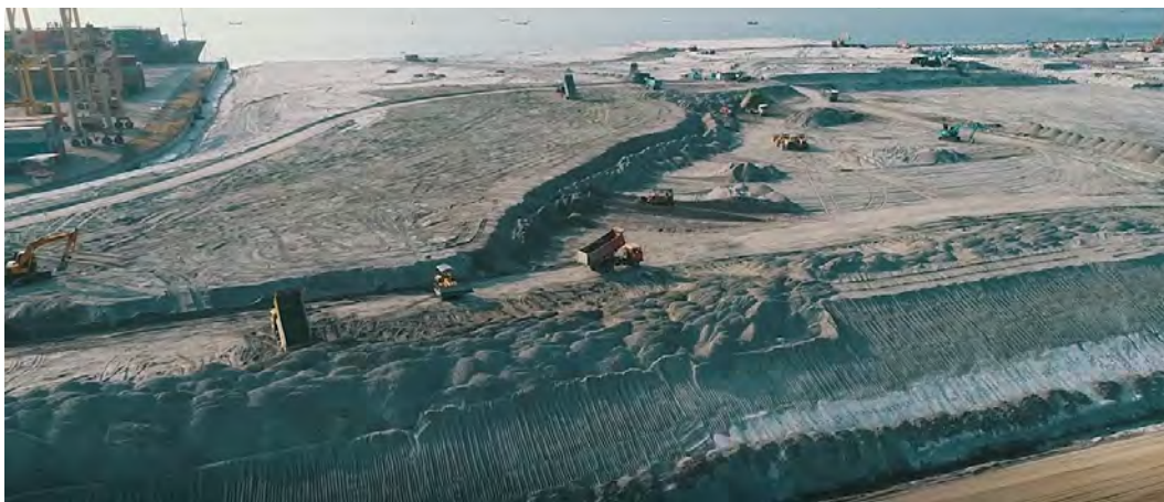
Gambar : Cutting Preloading
