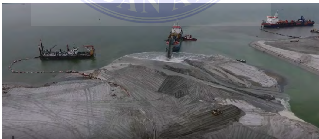
Gambar : Reclamation Work
