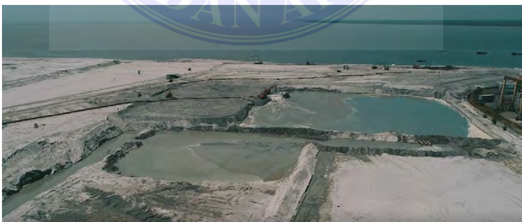
Gambar : Preloading Work
