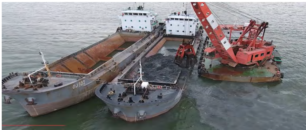
Gambar : Dredging Temporary Acces Channel
