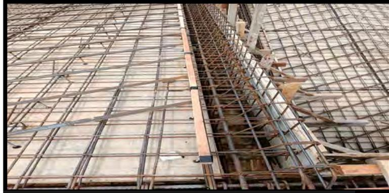
Gambar 4.3.2 bekisting balok
