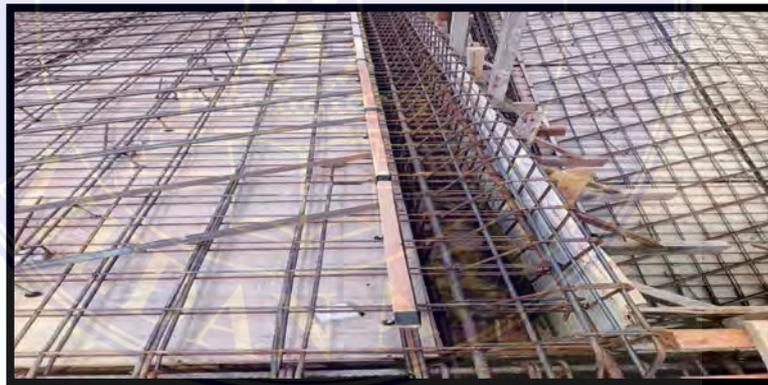
Gambar 4.3.2 bekisting balok
