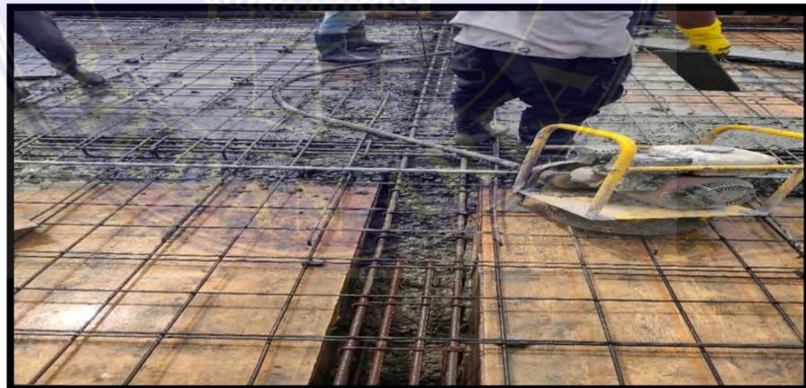
Gambar 3.1.7 Beton Vibrator
