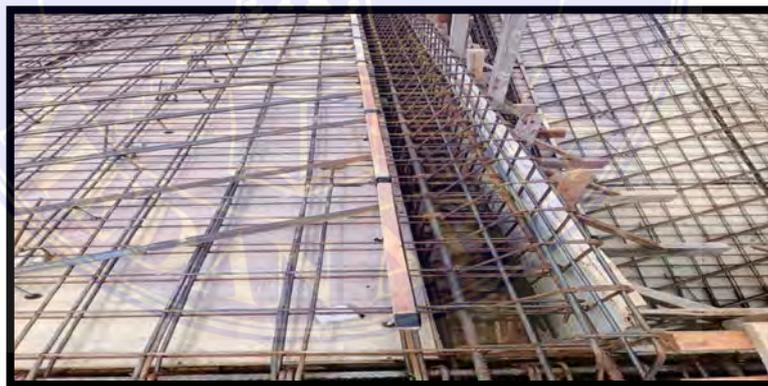
Gambar 4.3.2 bekisting balok
