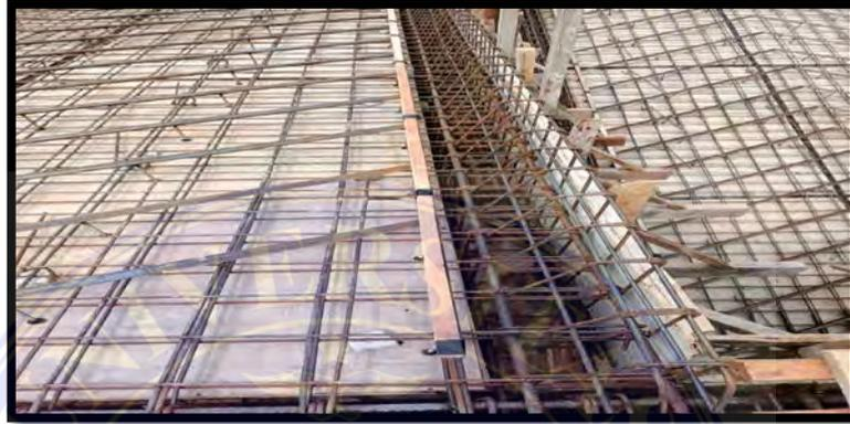
Gambar 4.3.2 bekisting balok
