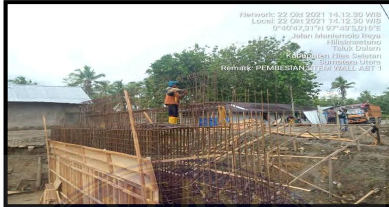
Gambar 4.2 Pembesian Dinding Abutment Segmen Kedua
