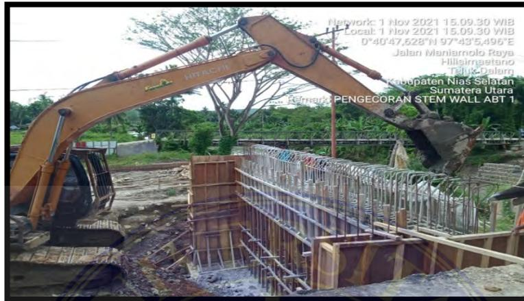
Gambar 4.7 Proses Pengecoran Abutment
