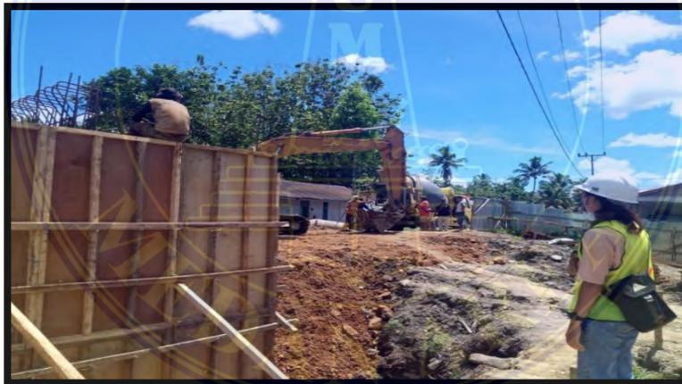
Gambar 4.8 Proses Pengecoran Abutment
