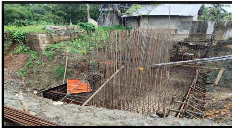
Gambar 4.1 Pembesian Dinding Abutment Segmen Pertama
