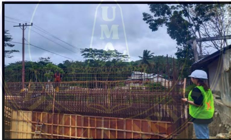
Gambar 4.3 Pembesian Dinding Abutment
