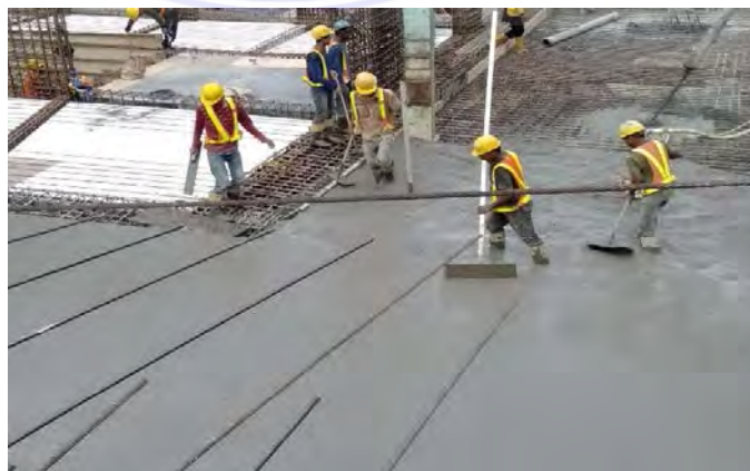
Gambar 4.9 Proses Perataan hasil coran
