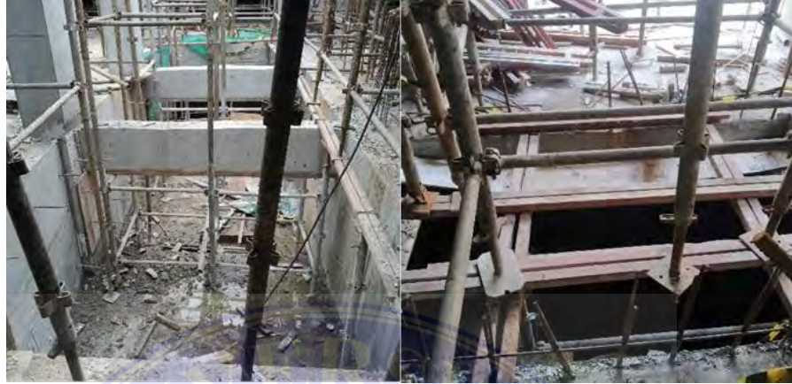
Gambar 3.5 Ground Water Tank
