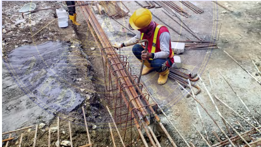
Gambar 3.4 Tie – Beam/sloof
