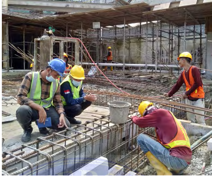
Gambar 4.5 Pemberian beton decking
