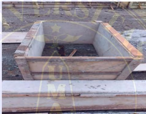
Gambar 4.10 Bekisting Pile Cap
