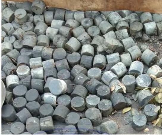
Gambar 3.13 Beton *Decking*
