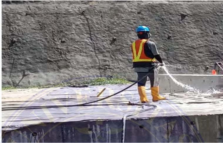
Gambar 4.56 *Curing beton*
