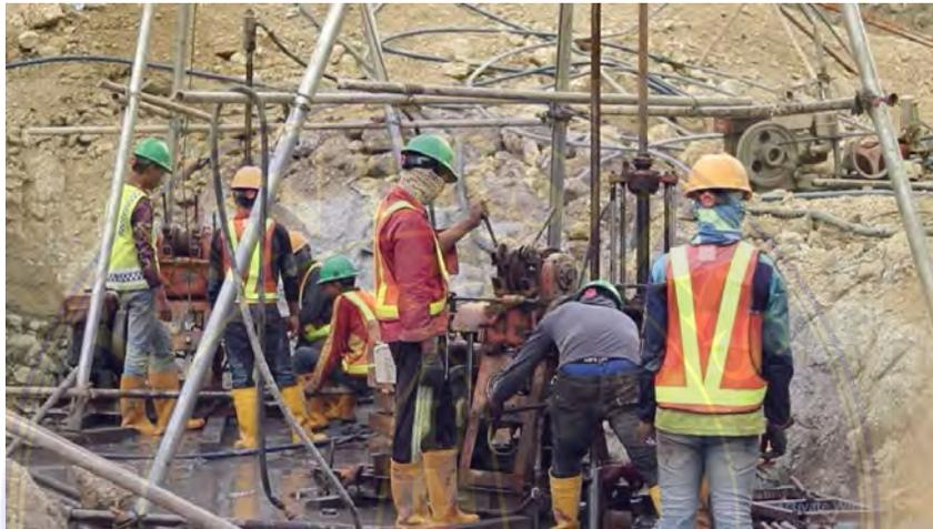
Gambar 3.30 Mesin Grouting
