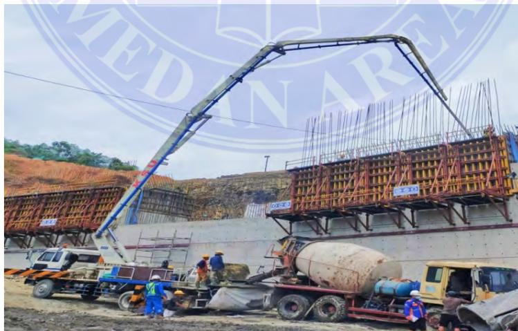
Gambar 3.18 Concrete Pump
