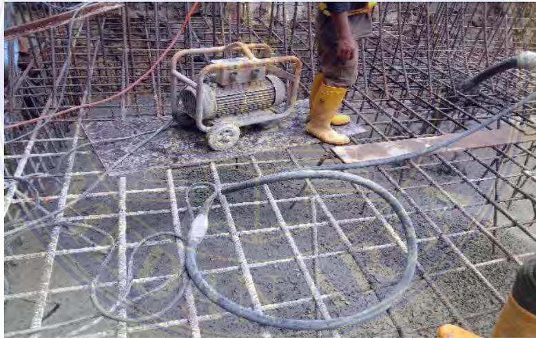
Gambar 3.10 Beton Vibrator
