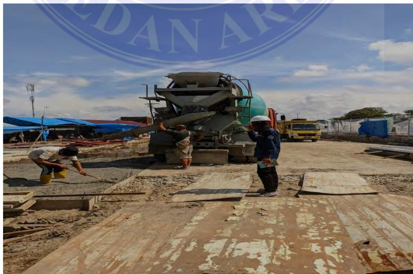
Gambar 3.11 Beton *ready mix*
