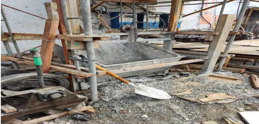
Gambar 3.20 *Concrete Bucket*
