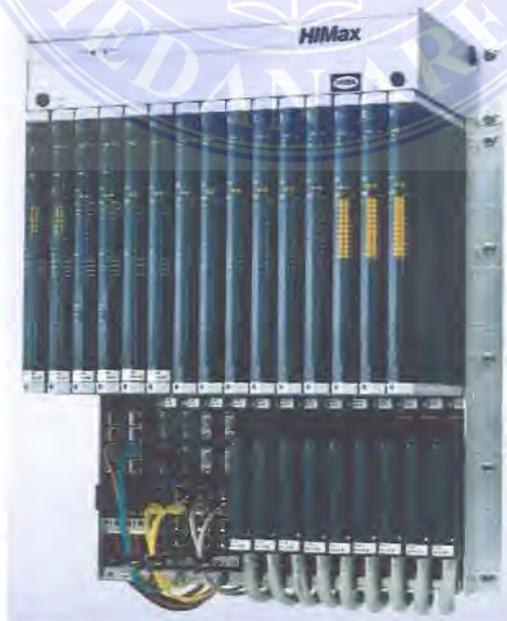
Gambar 2.3 Programmable Logic Control
