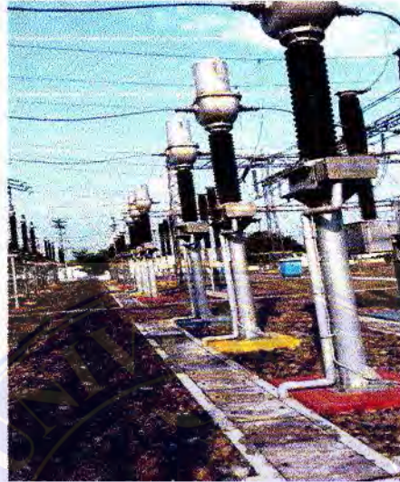
Gambar 3. Curren Transformer
