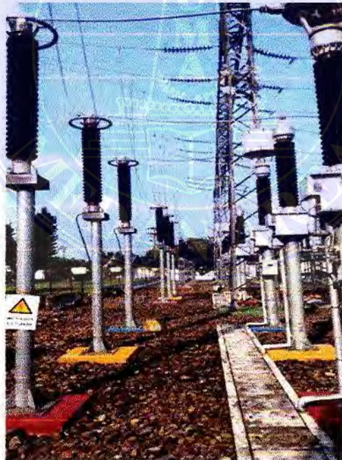
Gambar 1. Lightning arrester
