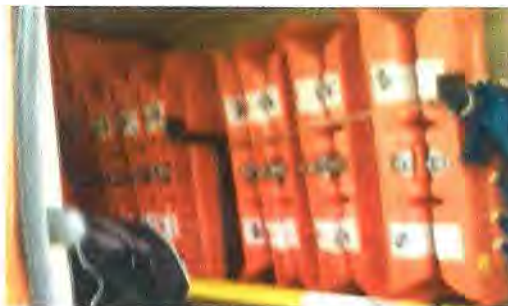
Gambar 2.12 Conductor Cover
