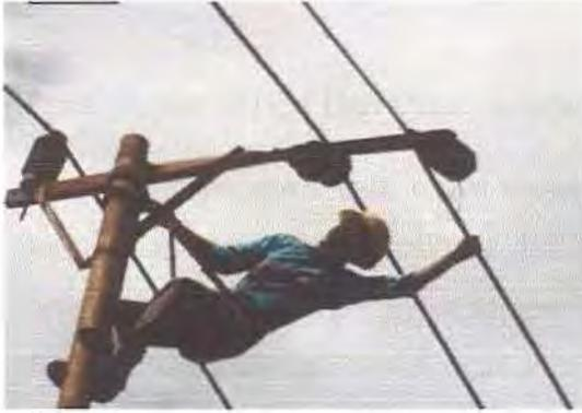
Gambar 3.7: Propes Penikan Kabel Sutm Yang Terlepas Dari Pin Isolator
