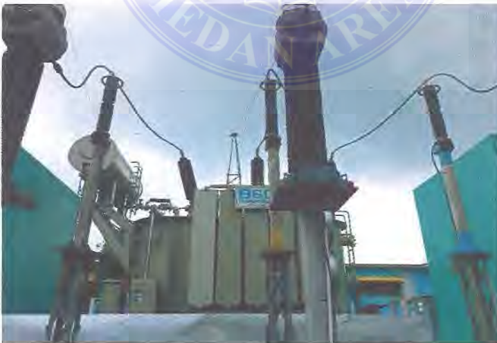
Gambar 5. Transformator Daya
