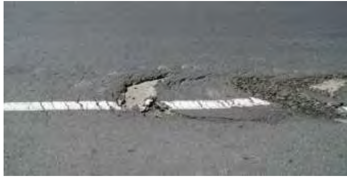
Gambar 2.18 Slippage Cracking
