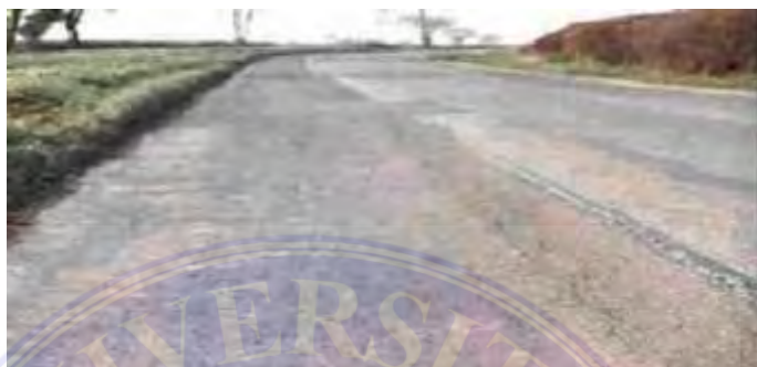
Gambar 2.9. Joint Reflection Cracking
