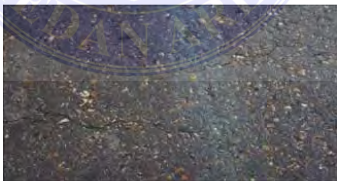
Gambar 2.13 Polished Aggregate Sumber : Dirjen Bina Marga 2017
