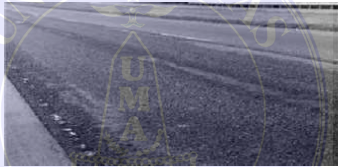
Gambar 2.20 Weathering and Ravelling Sumber : Dirjen Bina Marga 2017
