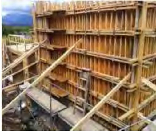
Gambar. 2.2 Bekisting semi sistem
