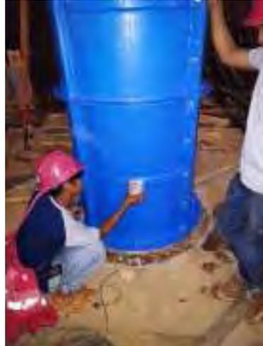
Gambar 2.6 Bekisting *fiberglass*
