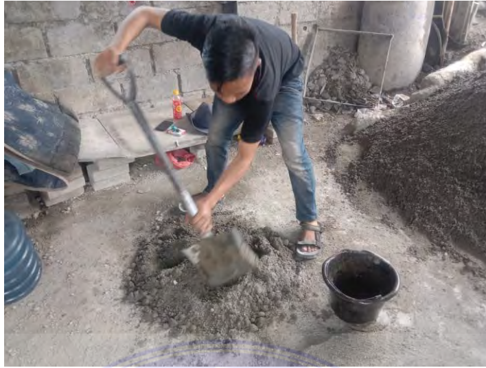
Proses pengadukan campuran paving block
