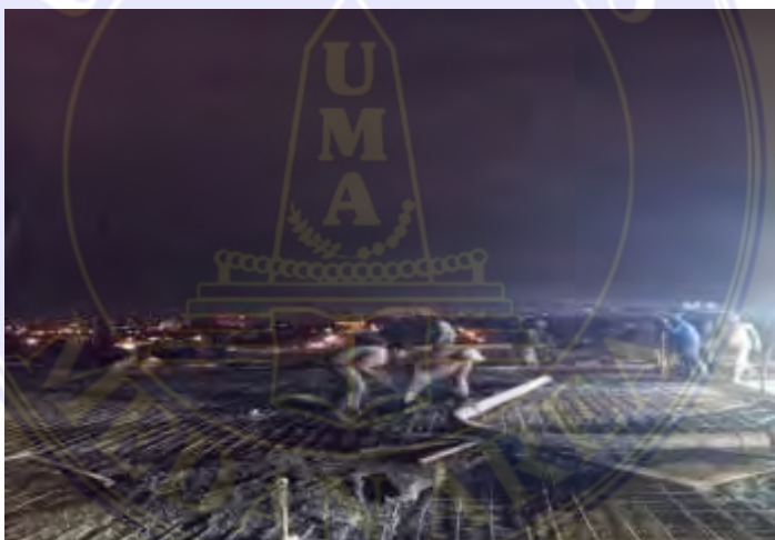
“Pengecoran Lantai”
