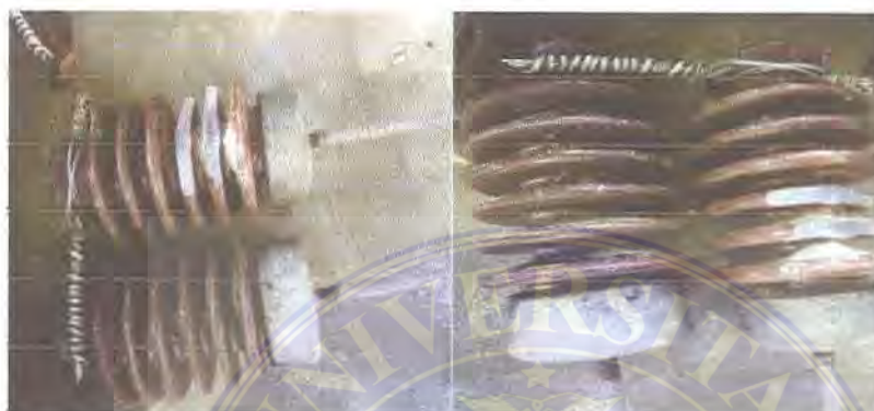
Gambar 3.1 Gangguan isolator pecah akibat flash over
