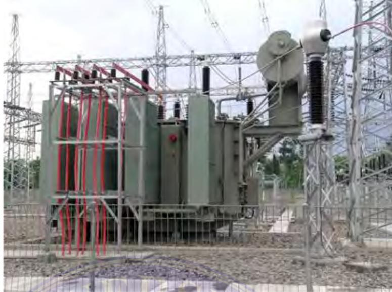
**Gambar 2.3 Transformator daya**
