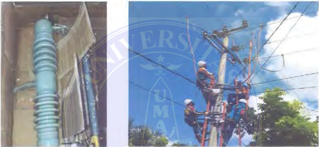
Gambar 3.2 : Fuse Cut Out (FCO)
