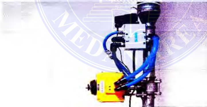
(Gambar 2.13 Selenoid Valve)
