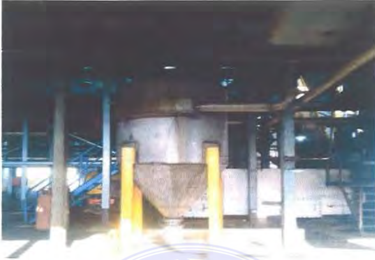
Gambar 3.18 Sand Trap Tank
