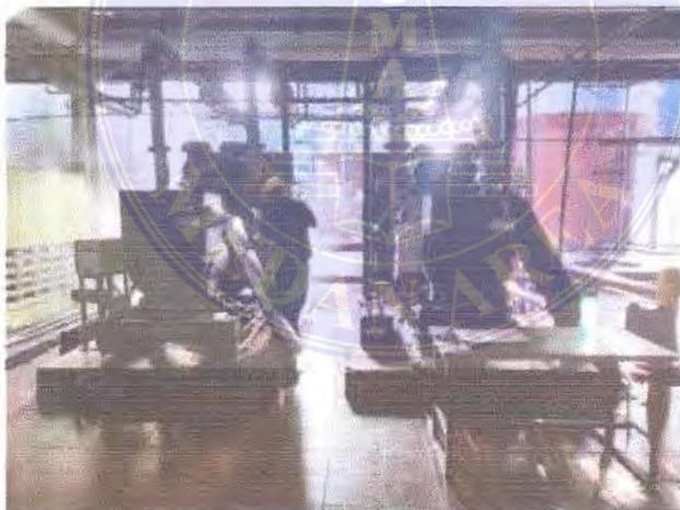
Gambar 3. 36 Mesin Diesel/Genset
