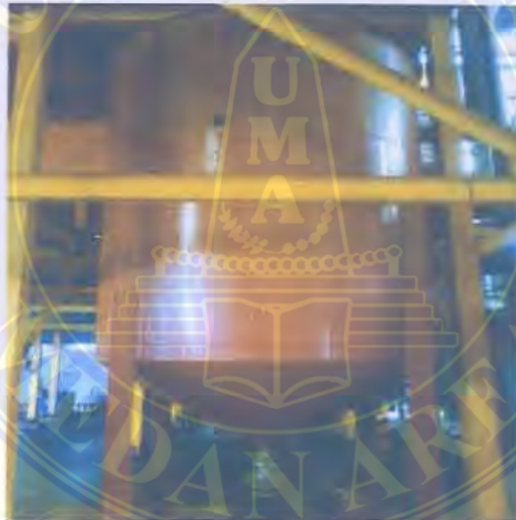
Gambar 3. 10 Sand Trap Tank
