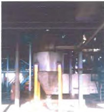
Gambar 3. 18 Sand Trap Tank
