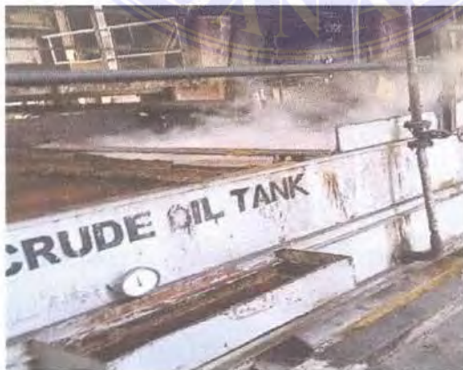
Gambar 3.18 Crude Oil Tank
